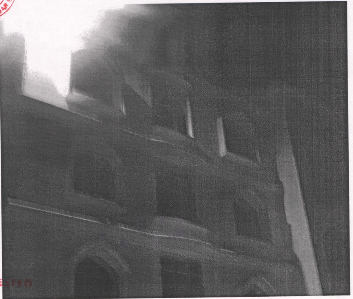
Rear view of the building
